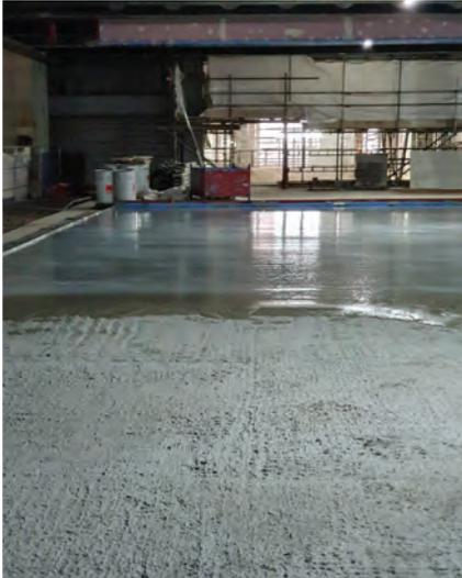
Installation of Cemfloor screed onto TLA insulated screed.
