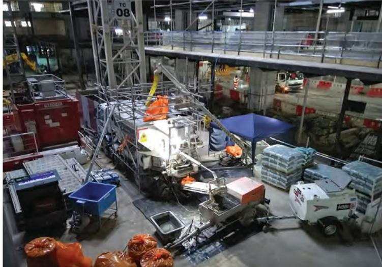
Bespoke volumetric mixing truck used to produce TLA insulated screed.
